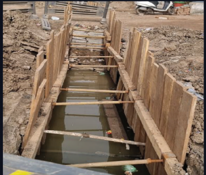
132 KV Torrent Power Gandhinagar line
