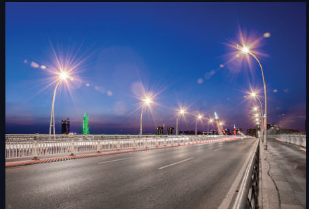
Street light work
