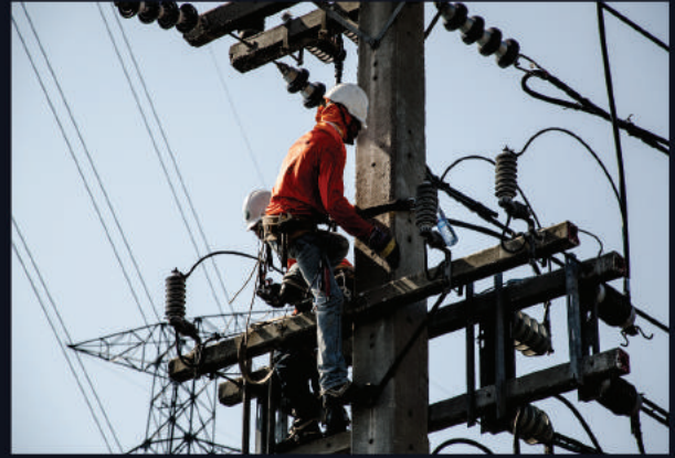
66/132/220 KV EHV line work and work of cable laying on tower
